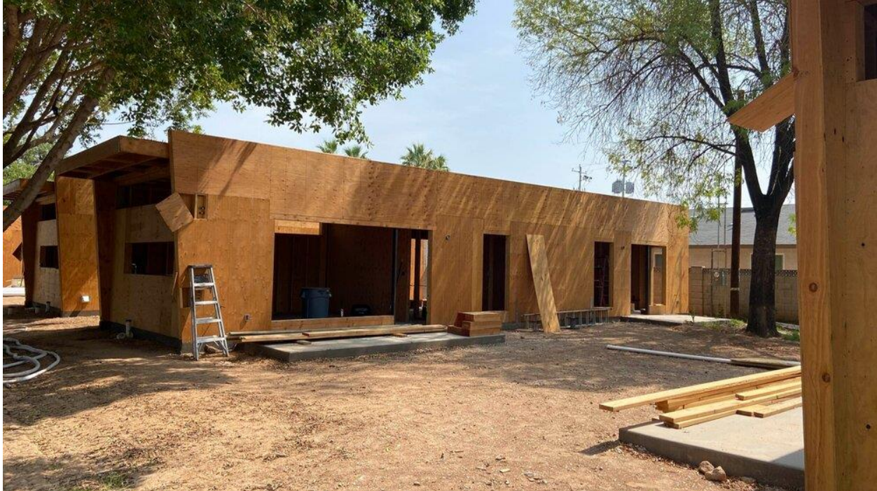
4Square detached fourplex under construction in Phoenix, Arizona. (Source: Venue Projects.)
